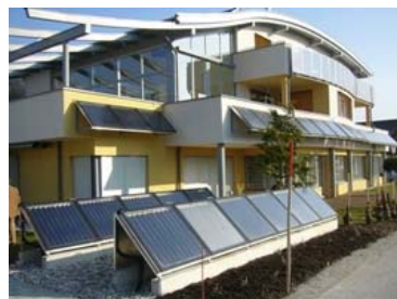
PSC10 Photo: Solarnext
